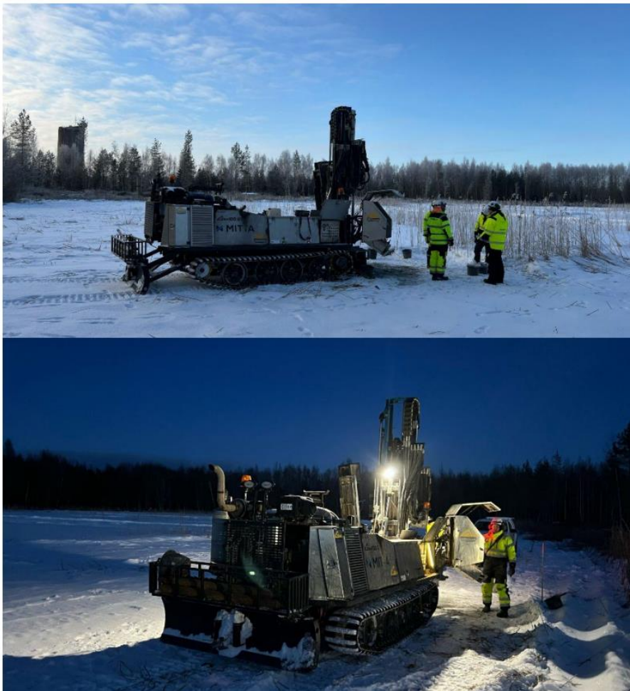
Drilling at the Korsnäs historic tailings storage facility (Source: www.prospech.com.au )
